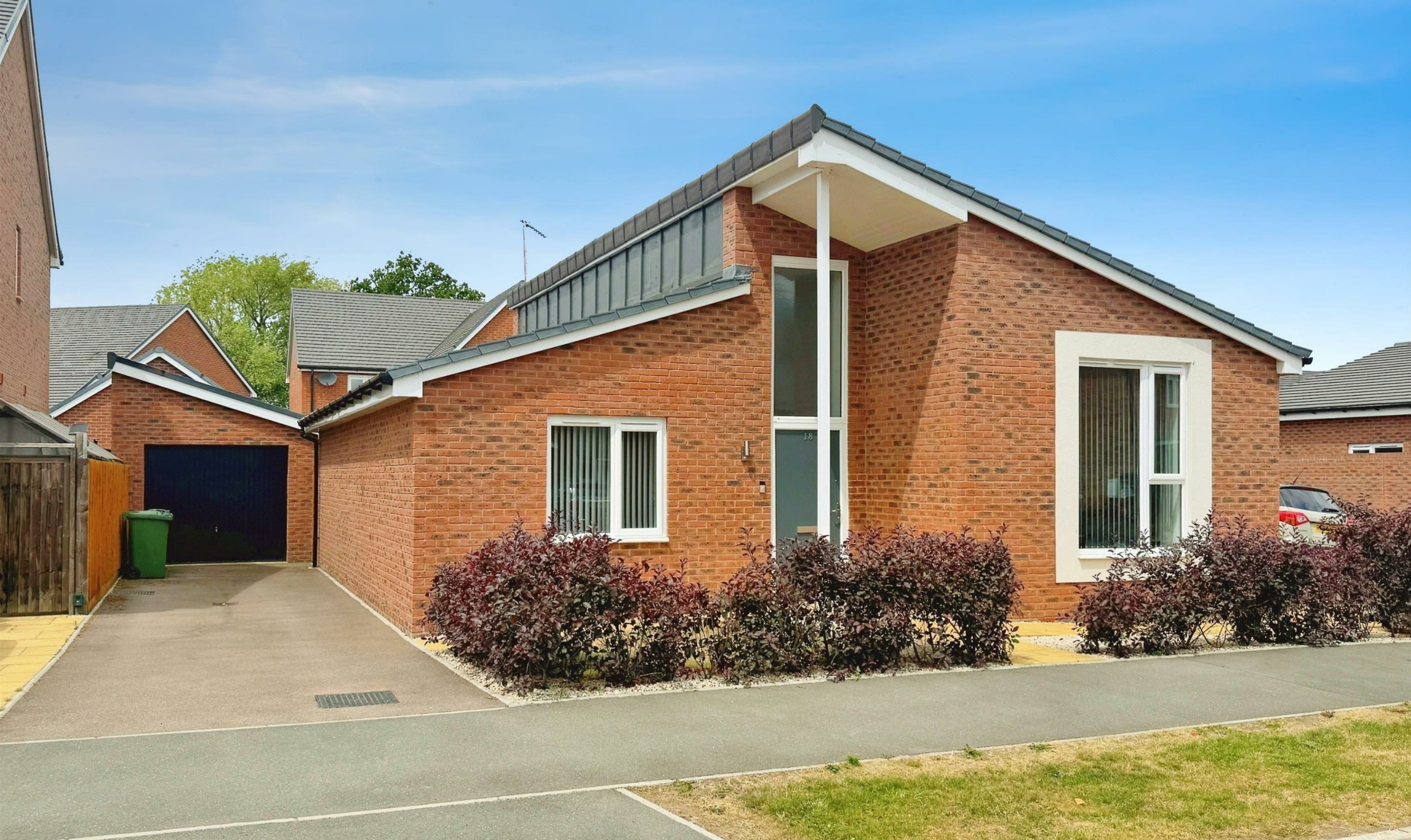
Poplar Drive , Meon Vale Stratford-upon-Avon, CV37 8FQ
